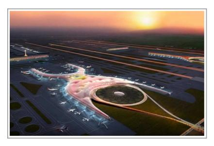
The architects are Sir Norman Foster and Fernando Romero. The entire terminal will be enclosed within a continuous lightweight gridshell, embracing walls and roof in a single, flowing form, evocative of flight.
